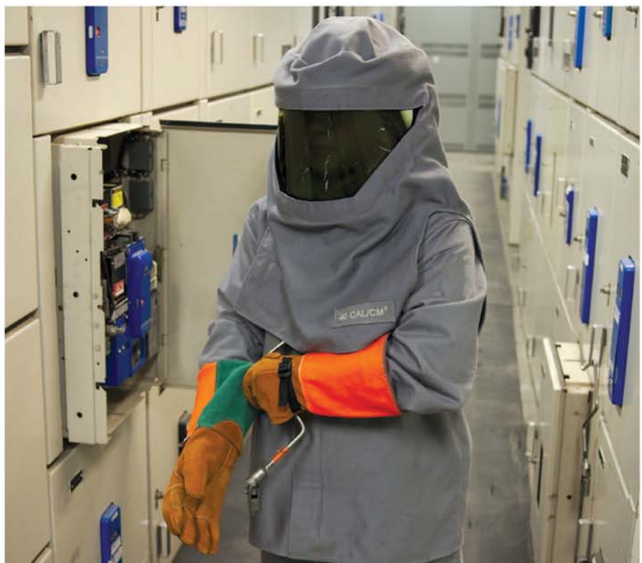
Abnormal conditions such as human interaction can lead to the breakdown in insulation of energized electrical equipment that can cause an arcing fault and an arc flash to occur.
